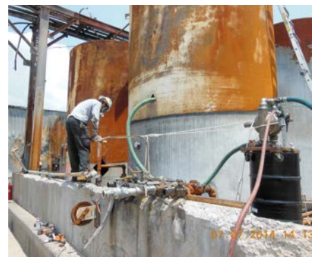
Tank Contents Removed Remotely Reduced PPE Requirements
