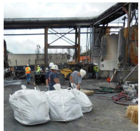
Spent Straw Filtration Barriers Placed in Supersacks of Disposal
