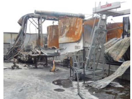
Tank Farm and Pipe Bridges Destroyed by Fire
