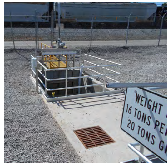
Weir Box with Automated Gate Installed at South Carolina Yard
