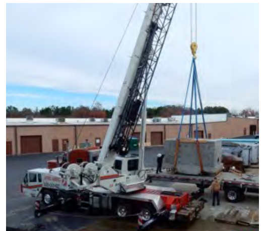
Precast Weir Box Lifted onto Flatbed Truck
