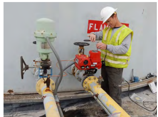
Automated Fuel Valve with Leak Detection Installed at Kansas City Yard
