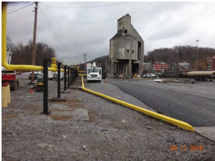
Construction of Road, Fuel Pipeline with Welded Secondary Containment & Supports, Curbing, and Concrete Rollover Curb
