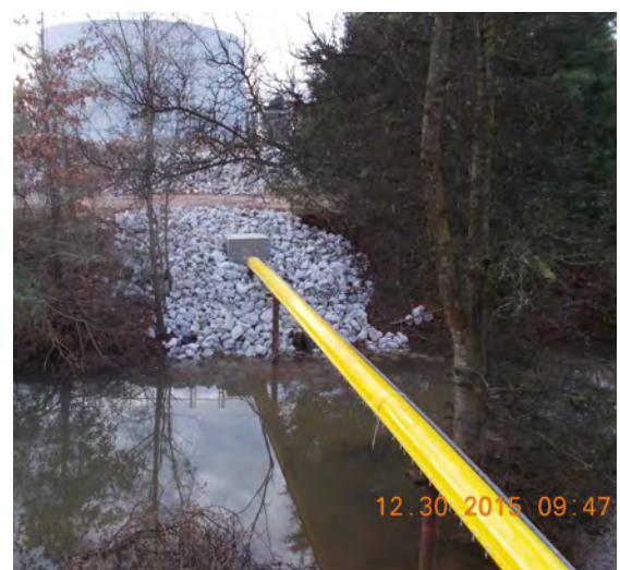
Containment Split Casing Installed On Fuel Line Crossing Stream in Alabama
