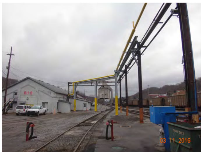
Overhead Pipe Supports & Split Casing Installed at West Virginia Yard
