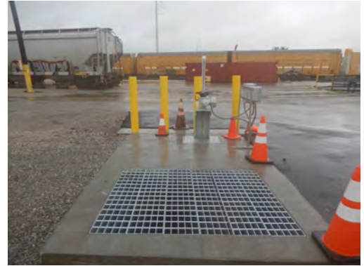
Weir Box with Automated Gate Installed at St. Louis Yard
