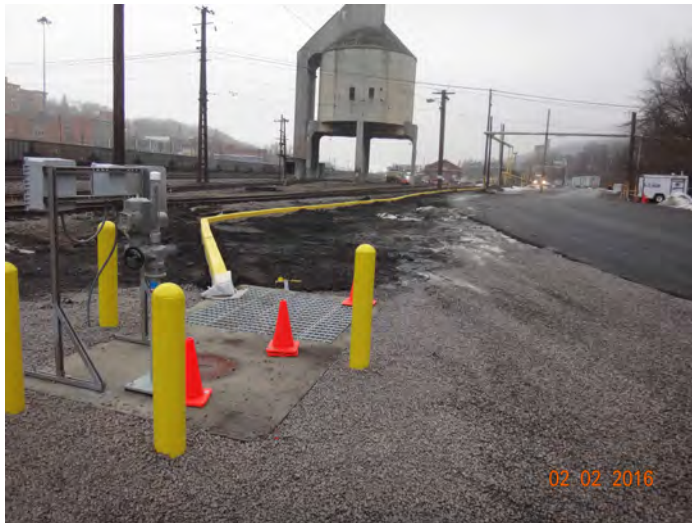
Weir Box with Automated Gate and Containment Wall Installed at West Virginia Yard
