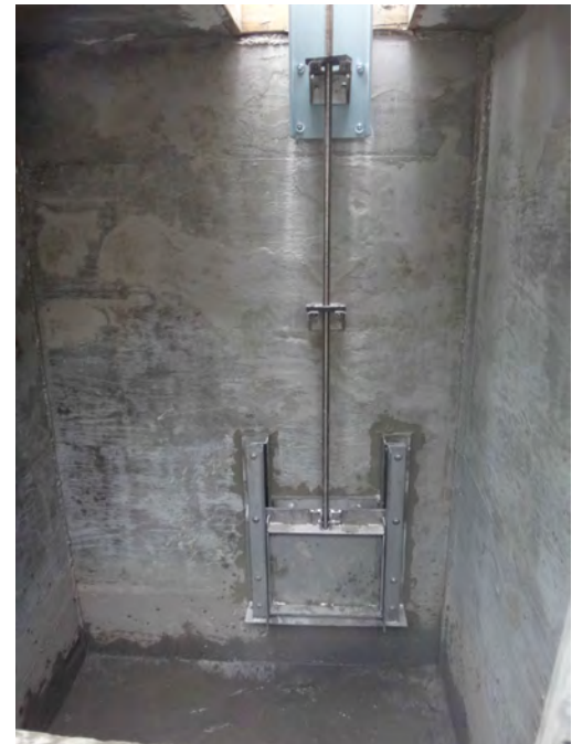
Sluice Gate Installed in Weir Box
