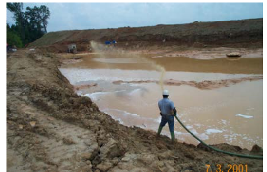
Application of HC-2000 to Surface Water & Sediment
