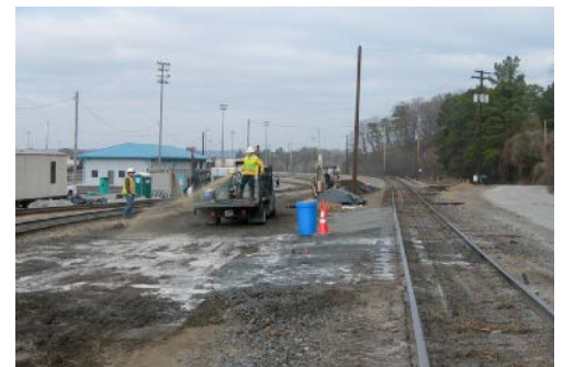
Residual Soil in Excavation Area Treated with HC-2000
