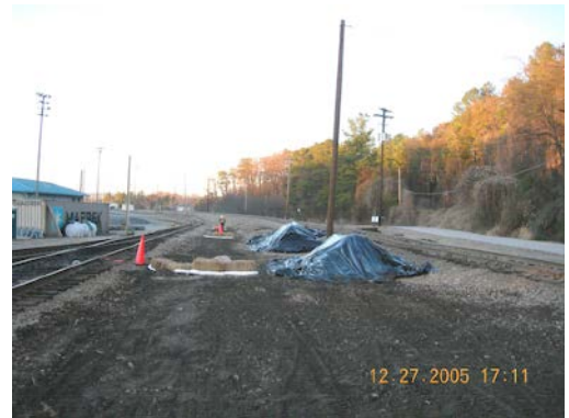
Excavated Fuel Saturated Soils Staged under Plastic
