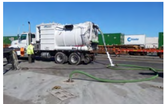
Two-Phase Vacuum Extraction removing Residual Diesel Fuel
