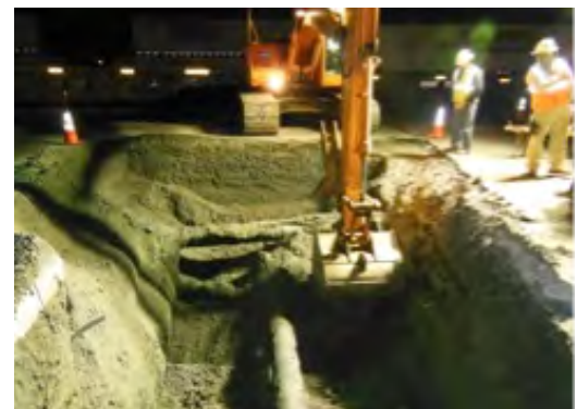
Leaking Fuel Line Located and Uncovered
