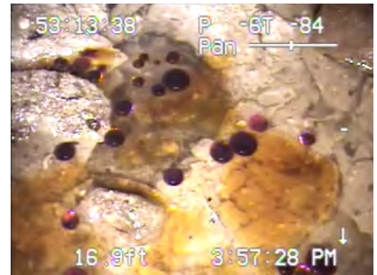
Stormsewer Fuel Infiltration Point Located by Remtech with CCTV Camera
