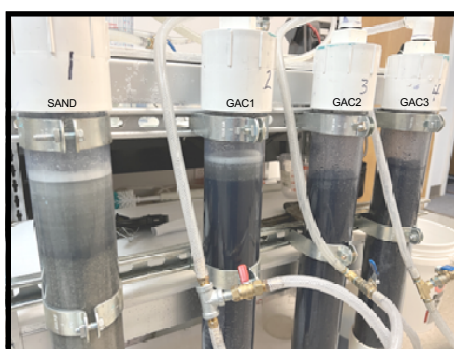
Figure 5: PFAS Foam Removed by 1st GAC Column
