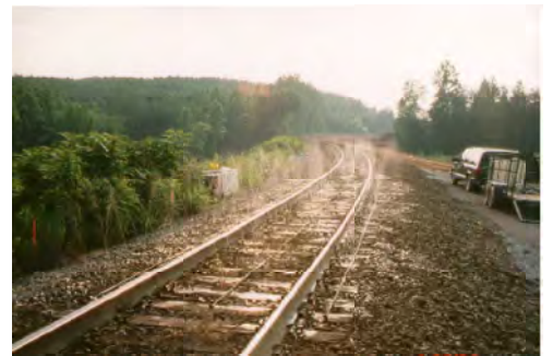
Mist Application Supplies Water & Oxygen to Site
