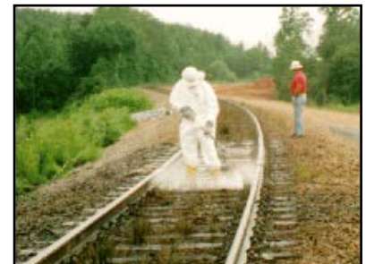
HC2 Degrades Diesel Fuel & Odors in Railroad Ballast w/o Track Time
