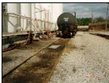
Motor Oil Contaminated Ballast Before HC2 Treatment
