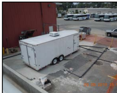
HC2 Removes Diesel Fuel in 10^{-6} cm/sec Conductivity Aquifer under Building
