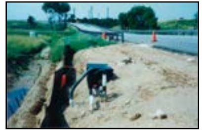
ATL Hartsfield Airport JP4 HC2 Remediation in Restricted Area
