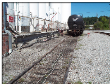
Ballast Staining & Oil Concentrations Reduced by 70%+ after 4 months of HC2 Treatment
