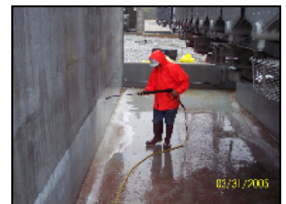
Transformer Oil Removed from Containment Structure at Power Plant
