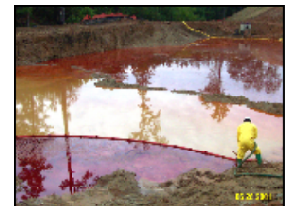
Bulk Diesel Removed prior to HC-2000 Treatment
