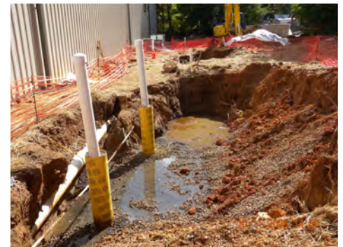
Interceptor Trench Installed Next to Building to Stop Fuel Infiltration
