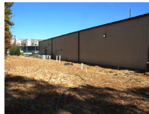
Completed Interceptor Trench with Recovery Wells
