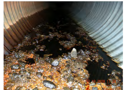
Culvert Draining Fuel from Contractor Facility
