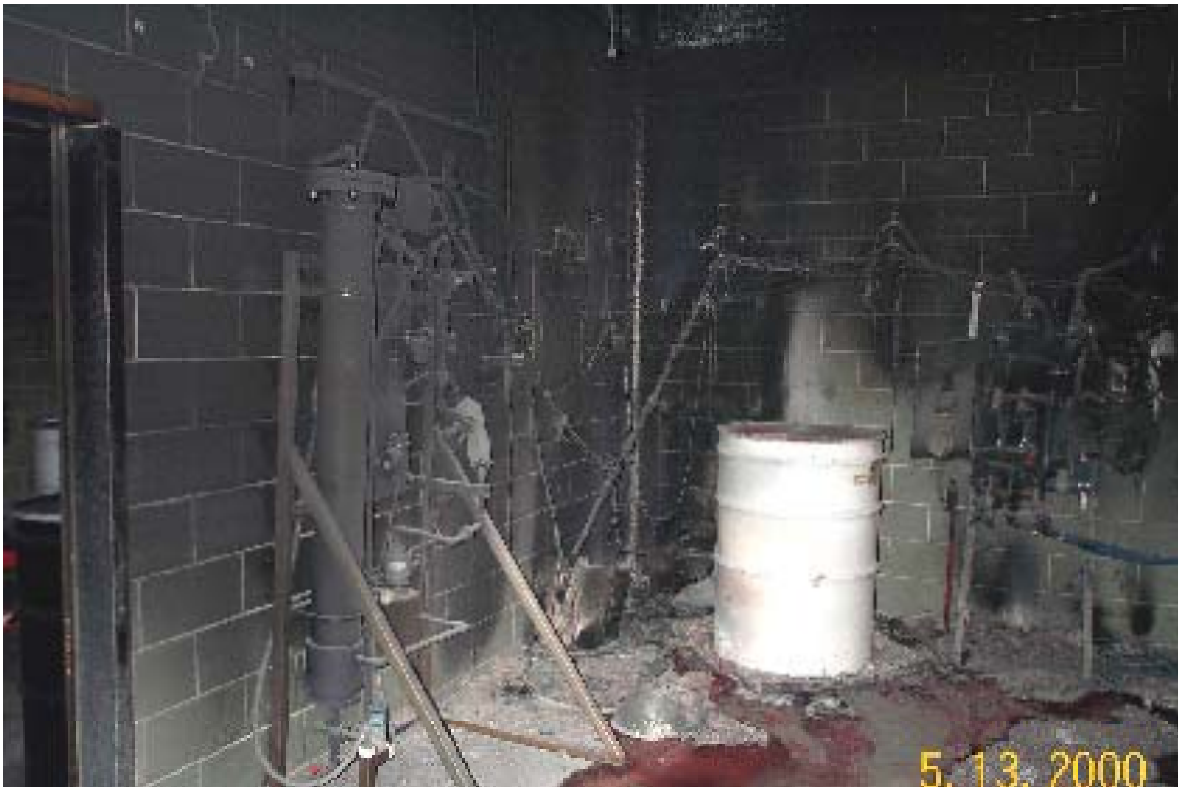
CASE 2-1: Chlorine dioxide generation system exploded in raw water pump building.
