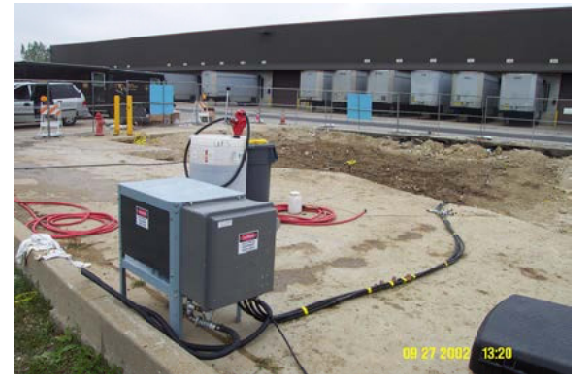
BioSparge Injection System at Freight Terminal
