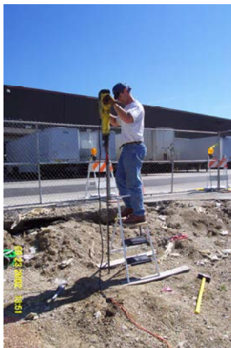
BioSparge Lances were Driven with Electric Jackhammer
