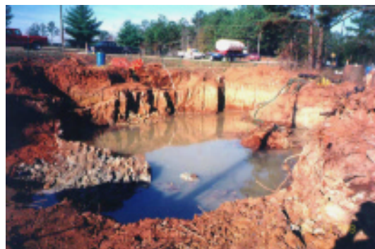
Excavation Following Removal of Saturated Soils
