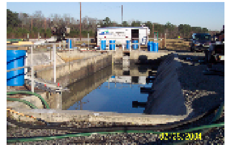
Kaolin Removed by Chemical Addition
