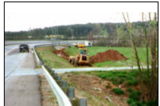
Ditch line Soil Removed to Biobed
