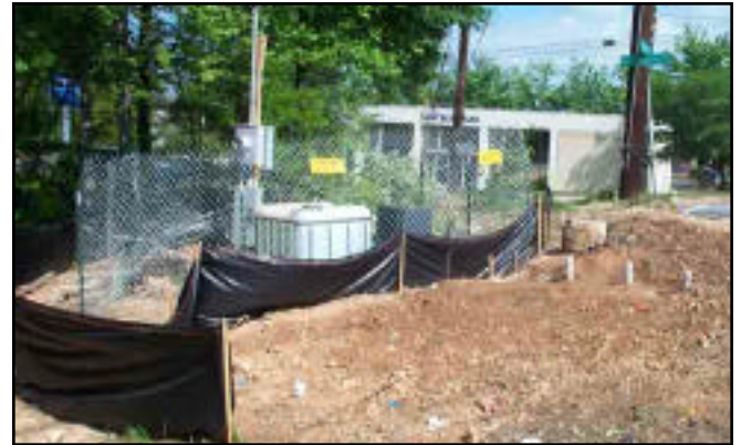
HC-2000 Injection Around Water Mains
