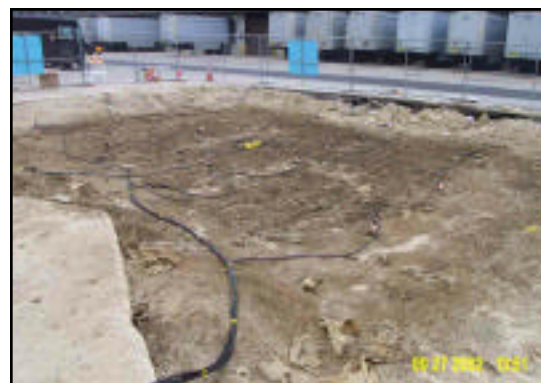
BioSparge Injection Grid
