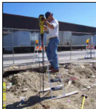
Sparge Tip Installation
