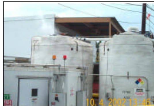
Collapsed Roof on Sodium Chlorite Tank
