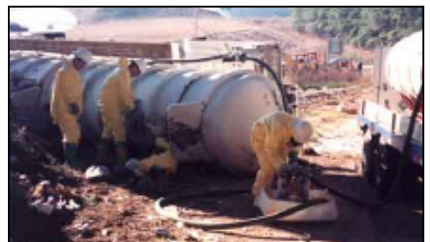
Acid Transferred with Poly Diaphragm Pump
