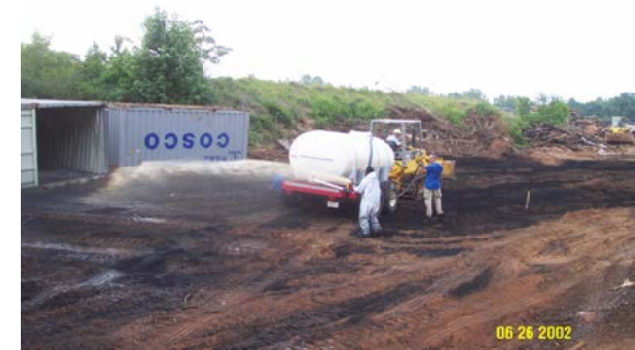
Carbon, Lime, and HC-2000 Odor Control
