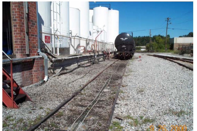
Rail Siding Following Four Months of Treatment
