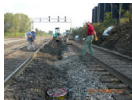
Leachate Collection System Installed between Two Mainline Tracks
