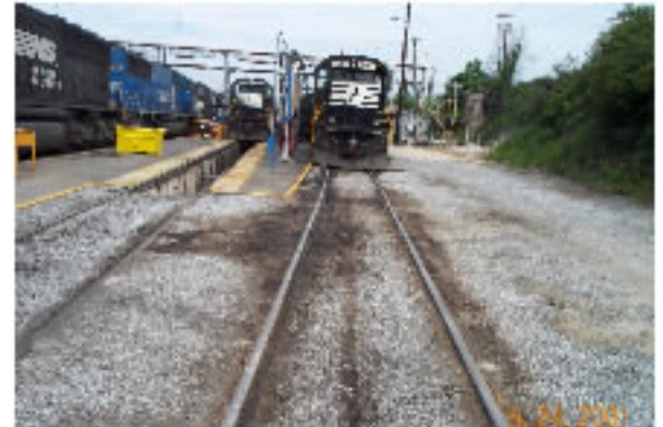
10 to 30% Ballast Stain Reduction During Test Period
