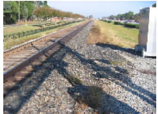
Ballast Stained by Diesel Fuel Release
