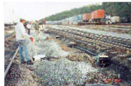
Leachate Collection System Installed
