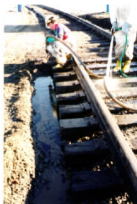
Lube Oil Desorbed from Ballast with HC-2000 and Pumped to Oil Water Separator
