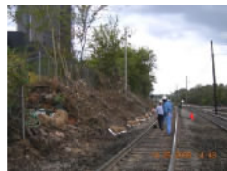
Straw Bale & Sorbent Boom Leachate Control System
