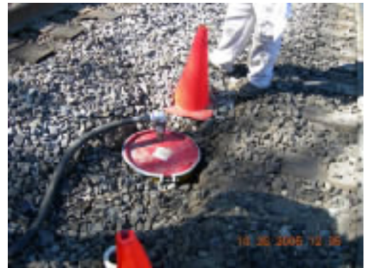
Leachate Sump Between Mainline Tracks
