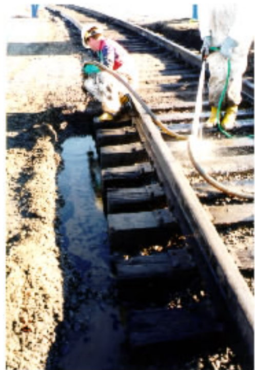
Lube Oil Flushed from Ballast with HC-2000
