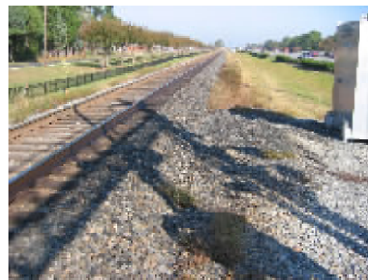
Diesel Stained Ballast from At-grade Lowboy Collision
