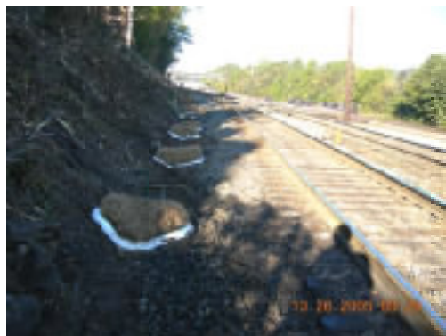
Leachate Collection System in Ditch
