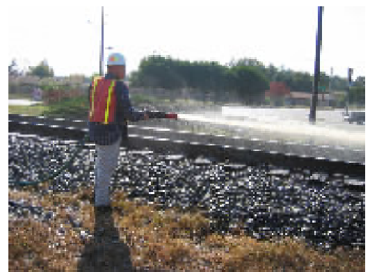
HC-2000 Applied with Fire Nozzle
