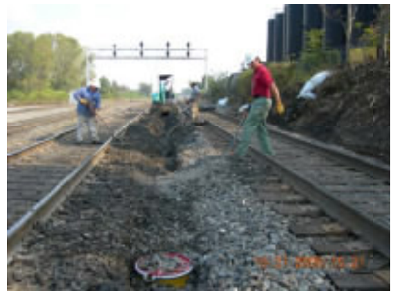
Installation of Drain Pipe & Sump
