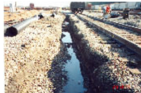
Diesel Fuel Collects in Trench for Leachate Control Pipe
